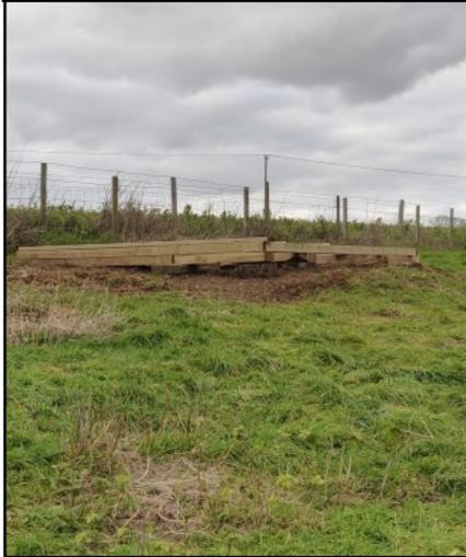
Although it hasn't been exactly goat shed building weather, our hardy band of volunteers has been undeterred. The ground has been dug away at the site of the new shed, and a sturdy base of reclaimed railway sleepers installed with a basic framework for the floor. During the last week or so, the uprights have been cut correctly (remembering before to measure twice of
